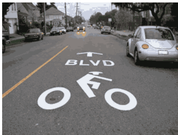
Figure 19. Bicycle boulevard pavement markings and signs used by the City of Berkeley. (source: Fehr and Peers)
