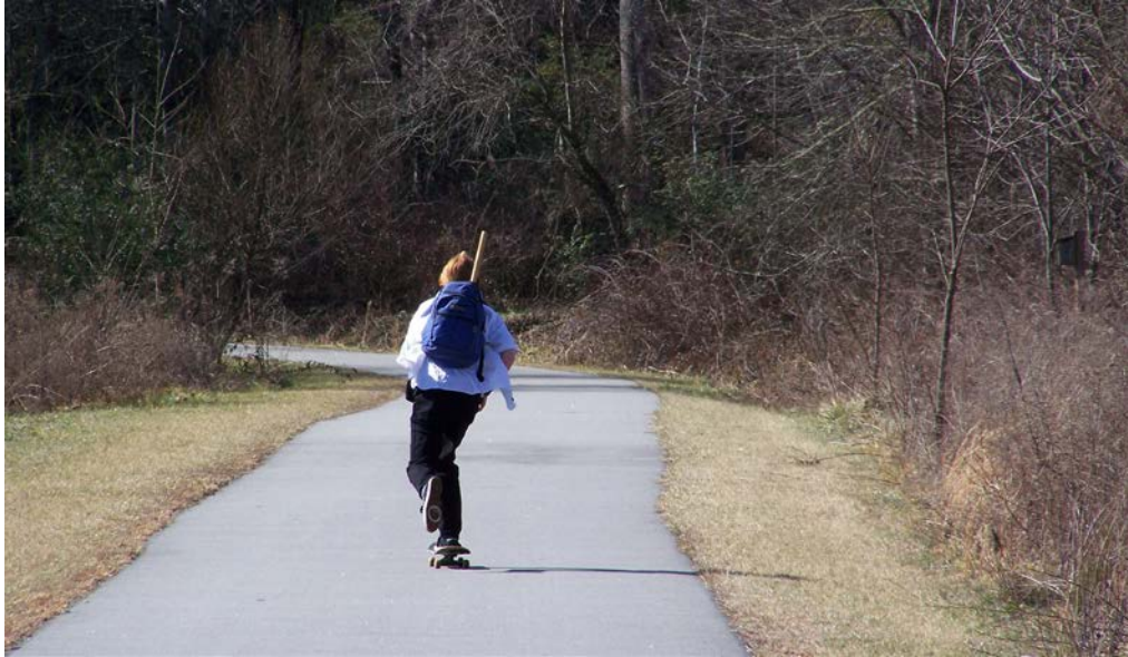
Figure 2. Path designed to include sufficient adjacent graded area and clearance from obstructions (source: www.pedbikeimages.org/Reuben E. Moore)
