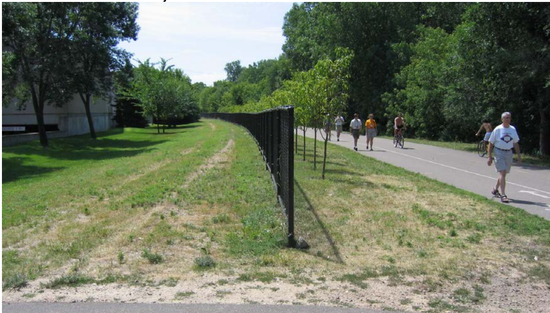
Figure 3. Bike path constructed in a former railroad right-of-way in Minneapolis, MN, where a portion of the right-of-way was reserved for potential future rail use.
