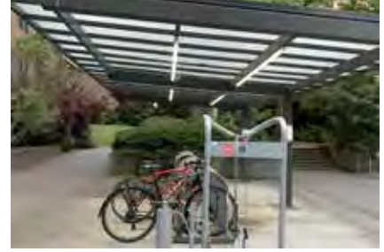
Racks under a shelter with lighting & repair station at UW (Photo: MIG/SvR)
