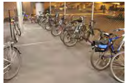
Racks do not provide 2 points of support (Photo: Alta Planning + Design)
