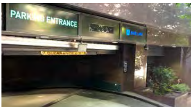
Parking garage with signed bike entrance over a delineated bike path (Photo: Alta Planning + Design)
