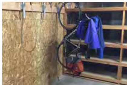
Anchoring and wood mounting is not theft resistant (Photo: MIG|SvR)
