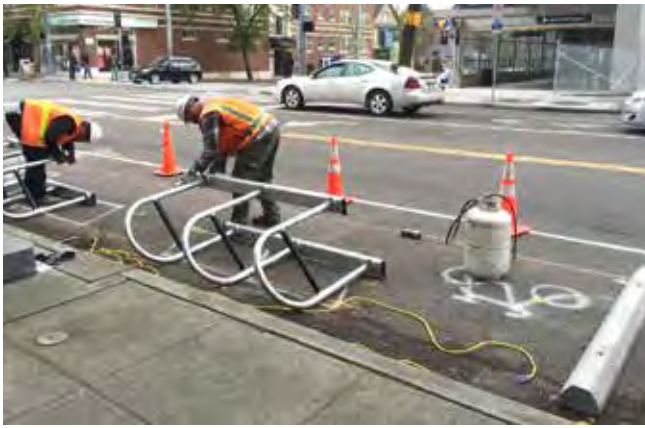
On-street bicycle corral installation at Capitol Hill Light Rail Station (Photo: SDOT)
