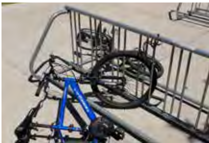
Rack does not provide 2 points of support or place to lock to frame (Photo: MIG/SvR)
